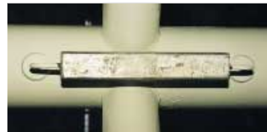
Corrosion protection – subsea paint system and anodes.
