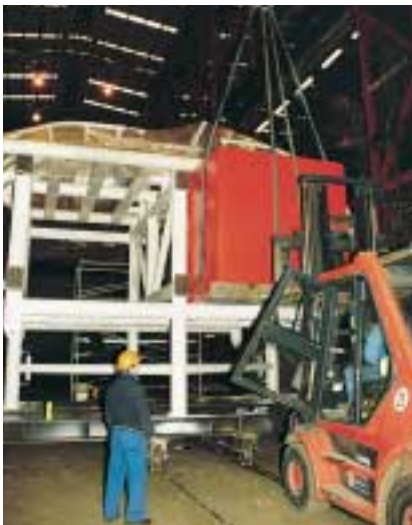
Buoyancy Elements being loaded into steel frame.
