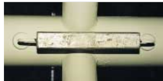
Corrosion protection – subsea paint system and anodes.
