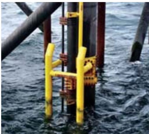
Riser Clamps installed on site
