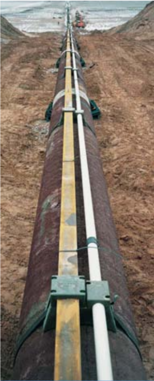
Piggyback Blocks installed onto onshore section of pipeline
