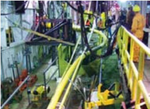
Piggyback Blocks being installed on Lay Barge
