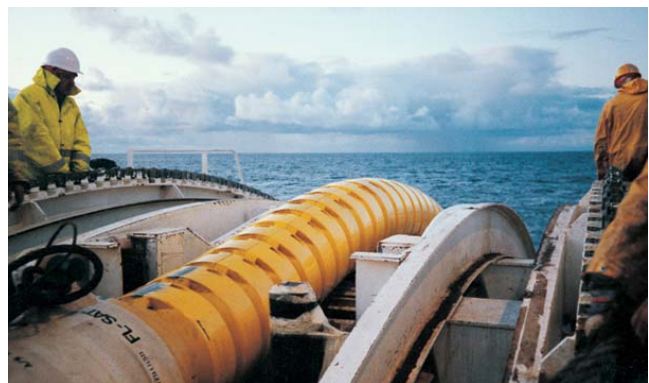
Overboarding complete Bending Restrictor
